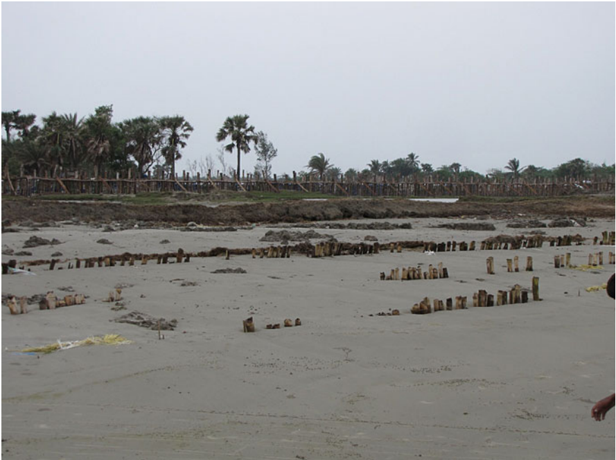
Succession of embankments due to erosion and poor hydrological conditions in river (Courtesy A. A. Danda)
