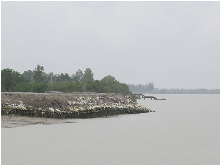
Endangered earthen embankment and jetty ghat due to caving of soil frequently encountered in the flood-prone areas (Courtesy D. Burman)
