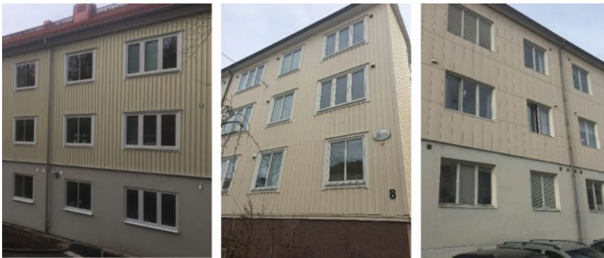
Fig. 2 Façade of Case A after the reconstruction of the wooden façade (left), Case B with unchanged façade (middle), and façade of Case C with the asbestos boards from 1970s (right)
