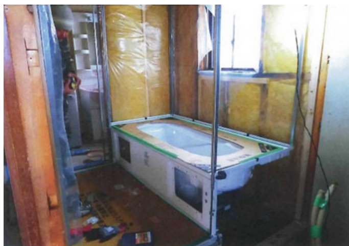
Fig. 4 Setting of new bathtub
