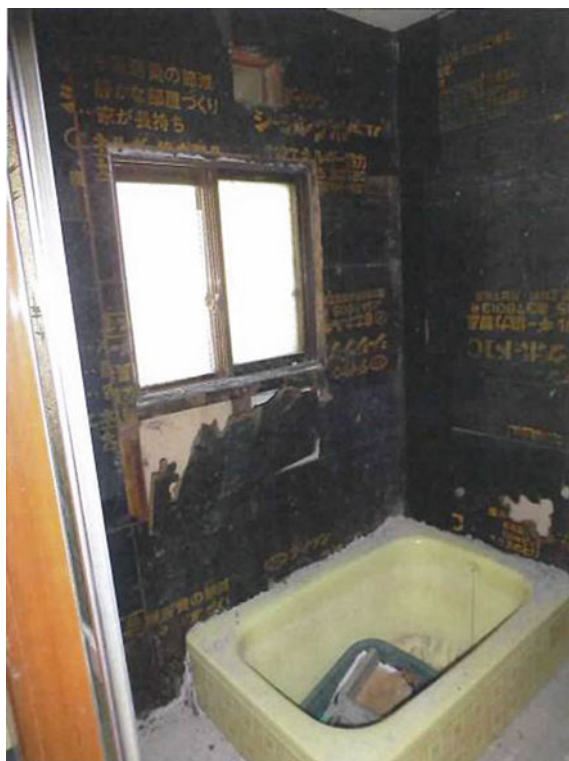
Fig. 3 Removal of inner finishing tile
