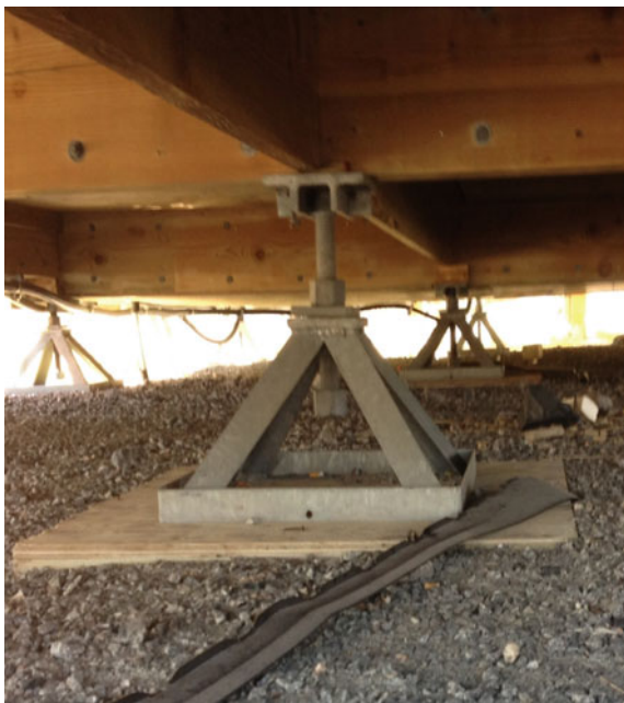
Fig. 2 Steel footing under wood beam
