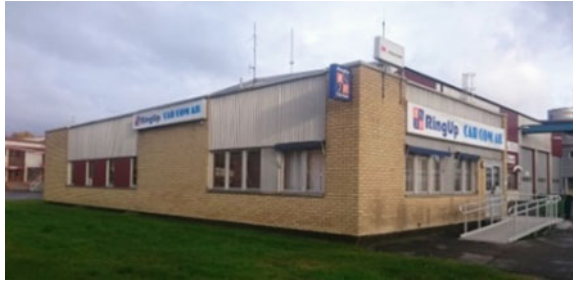
Fig. 1 Photo of the building before renovation, west and south wall
