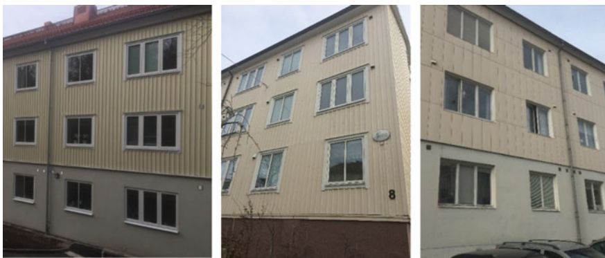
Fig. 2 Façade of Case A after the reconstruction of the wooden façade (left), Case B with unchanged façade (middle), and façade of Case C with the asbestos boards from 1970s (right)
