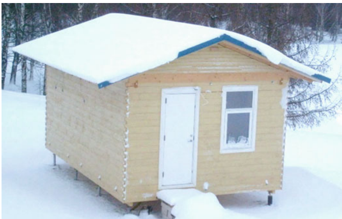
Fig. 1 Timber test house to investigate different insulation materials
