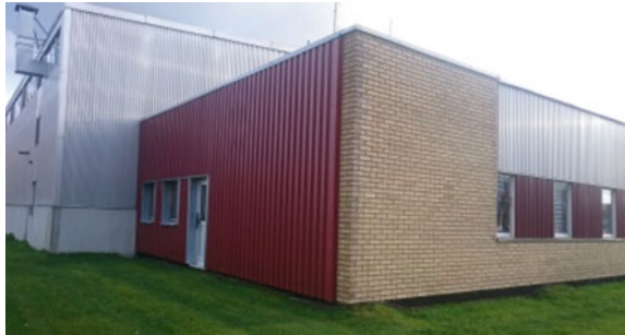
Fig. 2 Photo of the building before renovation, north and west wall
