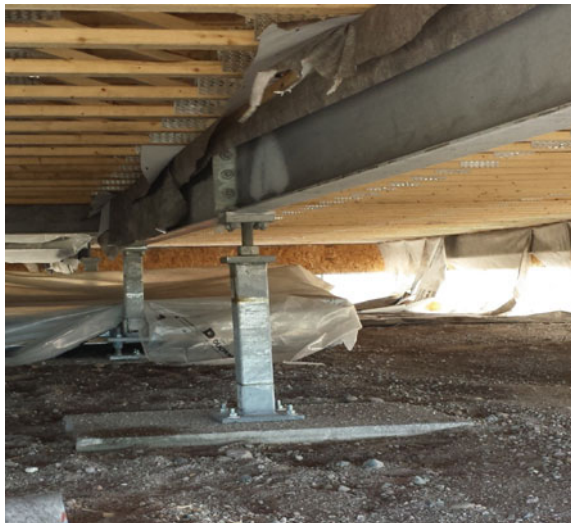
Fig. 1 Steel tripod footing
