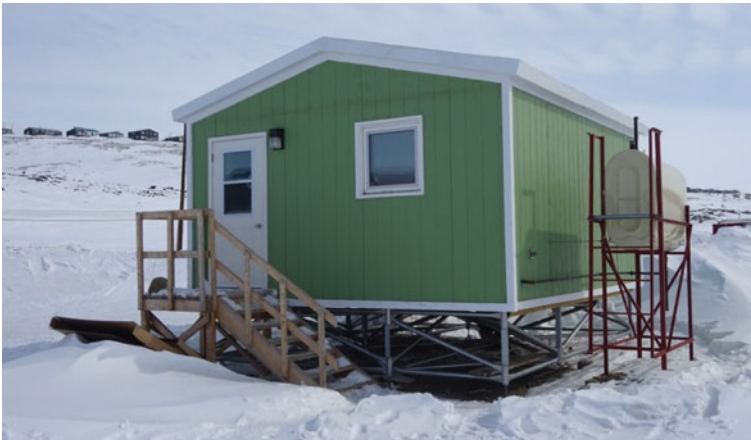
Fig. 1 Qikiqtaaluk demonstration house in Iqaluit
