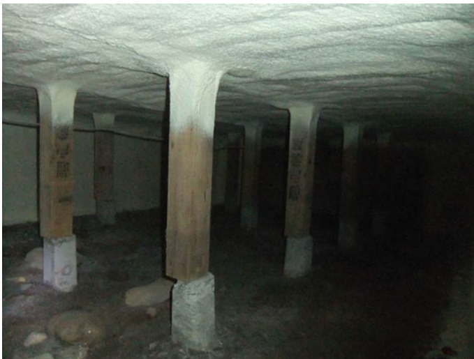
Fig. 6 Insulation of undersurface of floor
