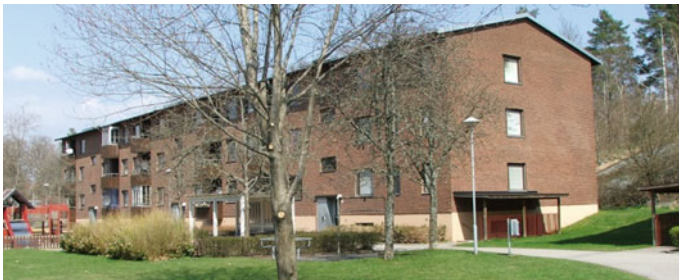
Fig. 1 The analysed concrete-frame building in Ronneby municipality, Sweden
