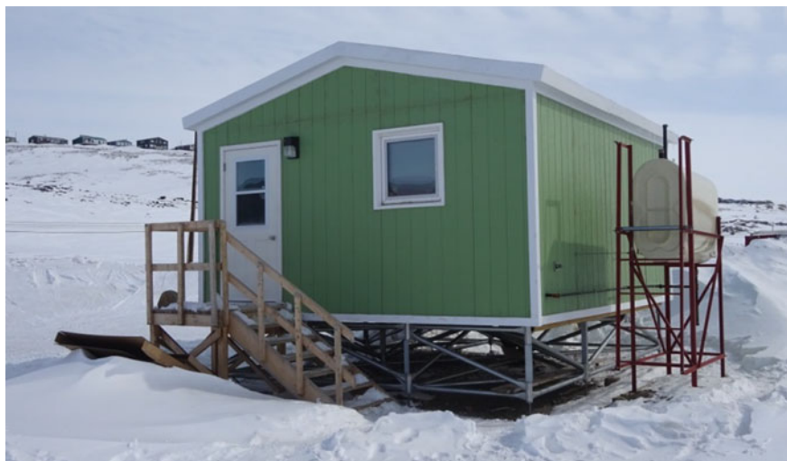
Fig. 3 Qikiqtaaluk demonstration house in Iqaluit
