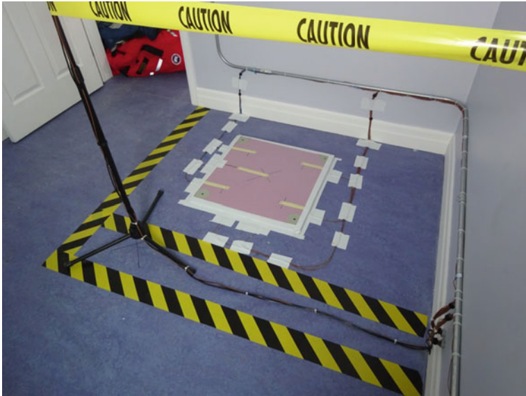
Fig. 4 Floor instrumentation module installed on site
