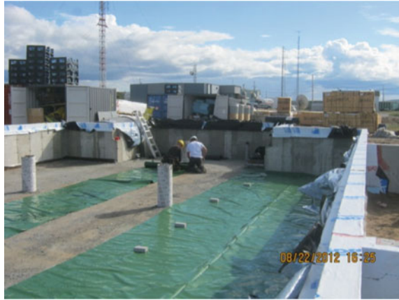
Fig. 3 Building basement in the North
