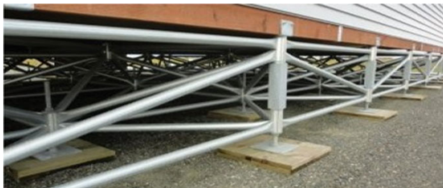
Fig. 4 Lattice structure under northern home
