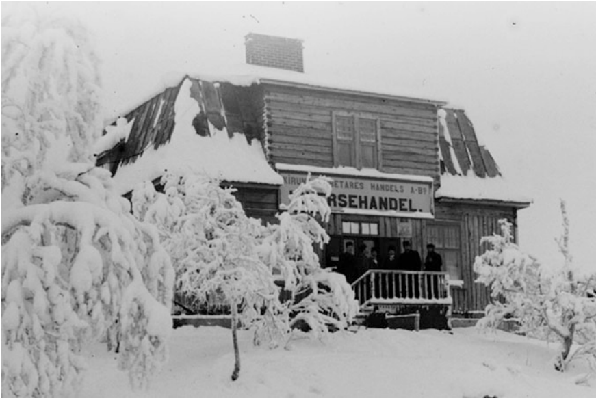
Fig. 5 Detail of a picture by Borg Mesch (© Kiruna Bildsamlingen) representing house B54 (ca 1901-02). Timber logs are disposed vertically on the bottom floor, horizontally in the attic
