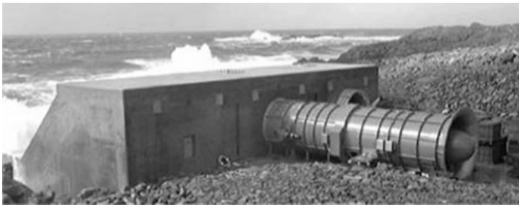
Fig. 2 Wave power station with oscillating water column
