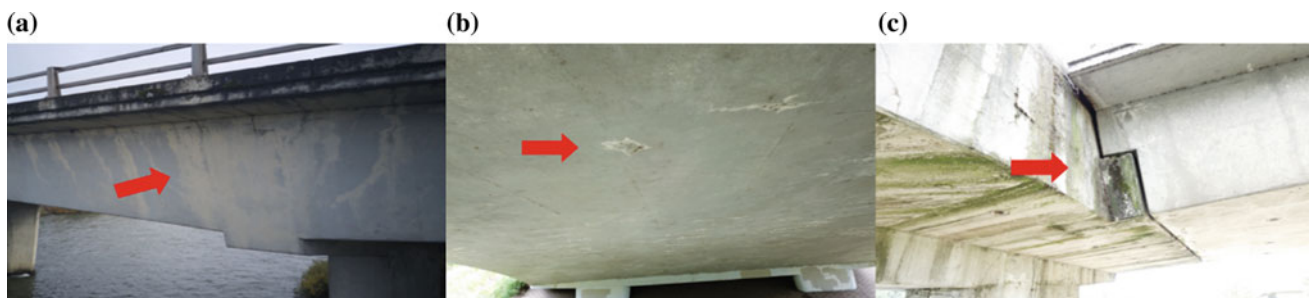
Fig. 74.3 Sample images of defects: a cracking with efflorescence on the side of the box b spalling area underside the box c rust staining on the concrete column
