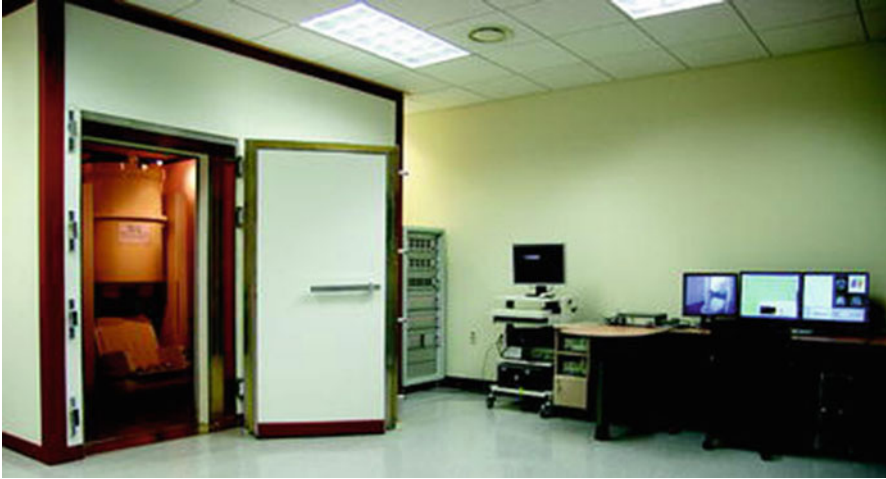
Fig. 11 A picture of a MEG system installed in a hospital. Helmet-shaped liquid He dewar mounted on a nonmagnetic gantry and inside a magnetically shielded room (MSR). Stimulation devices, acquisition, and analysis devices are outside the MSR
