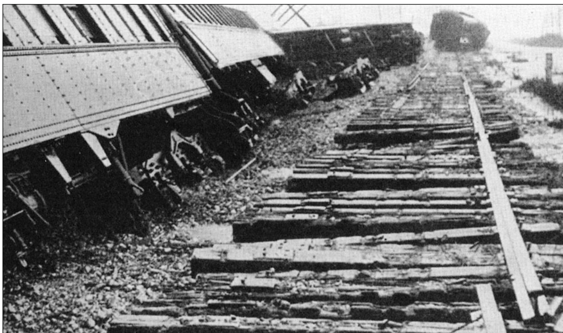
Fig. 4.16. A wrecked IC passenger train in Mississippi, resulting from a saturated roadbed that collapsed during the record 1937 flood. Note the high waters to the right of the roadbed.
