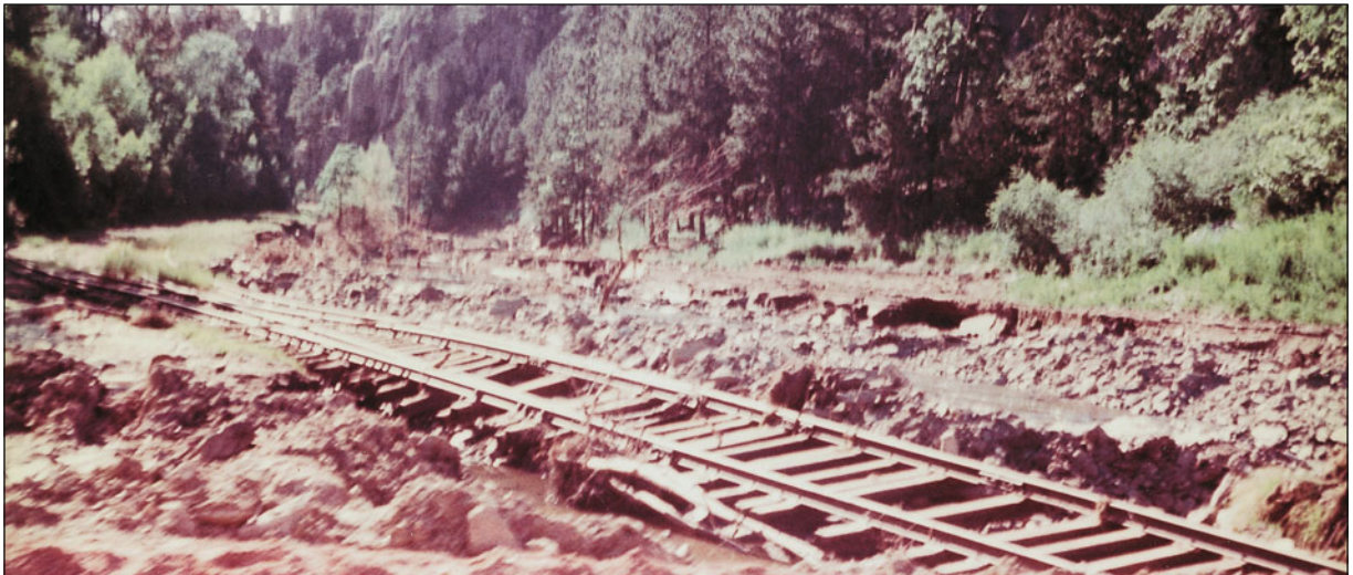
Fig. 2.7. A massive flash flood that originated in the Black Hills of South Dakota in July 1972 led to washouts of local rail lines, such as this one west of Rapid City.
