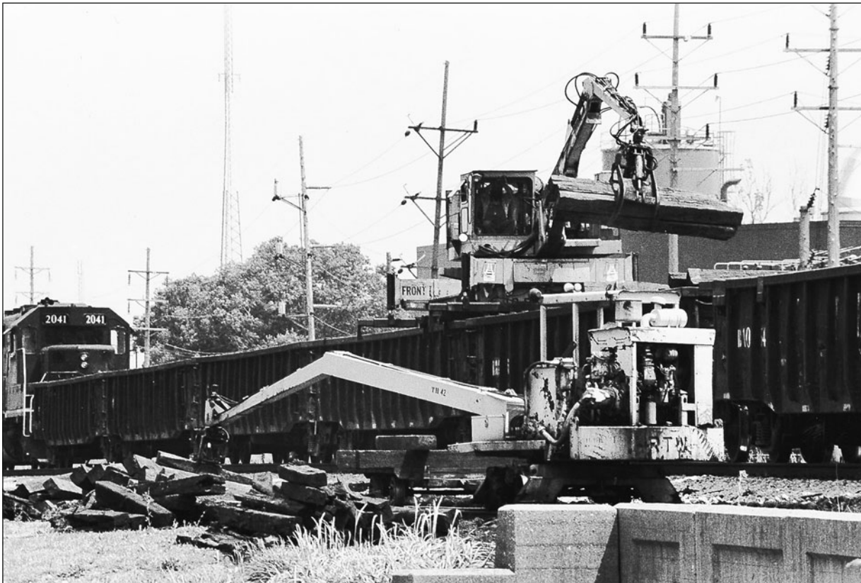
Fig. 5.12. Another weather-preventive action relates to care and maintenance of ties. Here an IC crew is removing and replacing aged ties.
