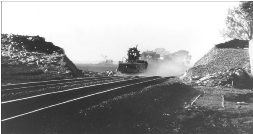
Fig. 5.18. A special levee was constructed across this UP line alongside the Mississippi River during the massive 1993 flood. A few days after the waters receded, a bulldozer is removing the rock and fill that crossed the tracks.
