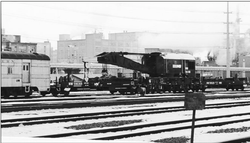
Fig. 5.14. A wrecker train is being assembled in the NS yards at Decatur, Illinois, to go to a snow-caused wreck and rerail the cars.
