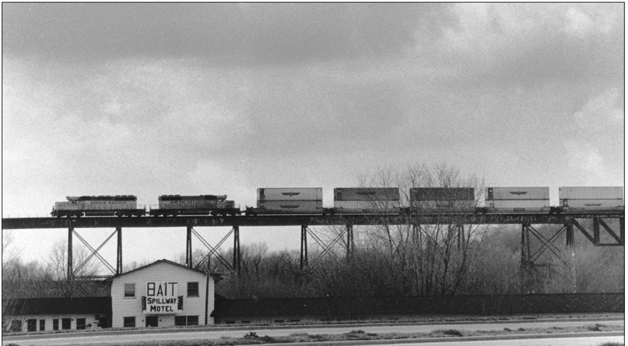
Fig. 4.32. Thunderstorms are developing as a southbound UP doublestack heads across a steel trestle in southern Missouri. Lightning struck the bridge a few minutes after the train passed.
