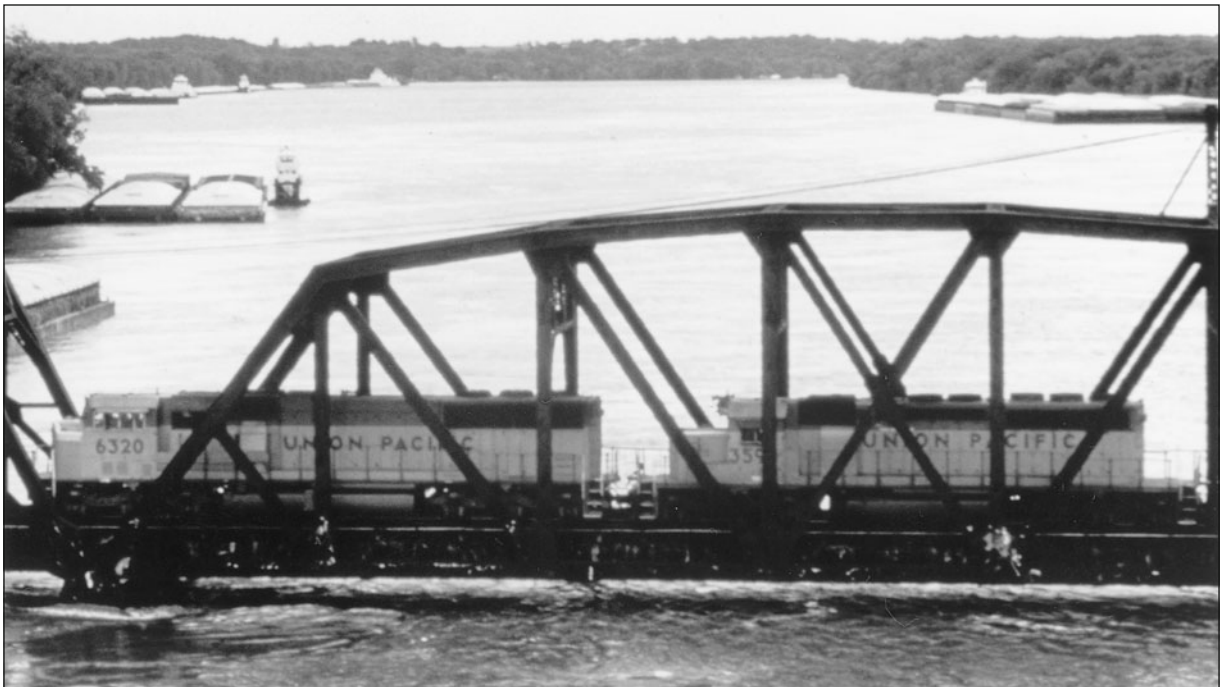
Fig. 3.9. A diverted UP train slowly crosses the still-operating bridge of the C&NW at Clinton, Iowa. Note the many barges anchored alongside the Mississippi River.
