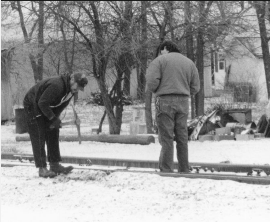
Fig. 2.19. Snow, ice, and cold weather freeze switches closed, unless heaters have been installed. Here two crew members of a grain train in a small Iowa town need to dig out a switch to an elevator service siding on a cold December day.
