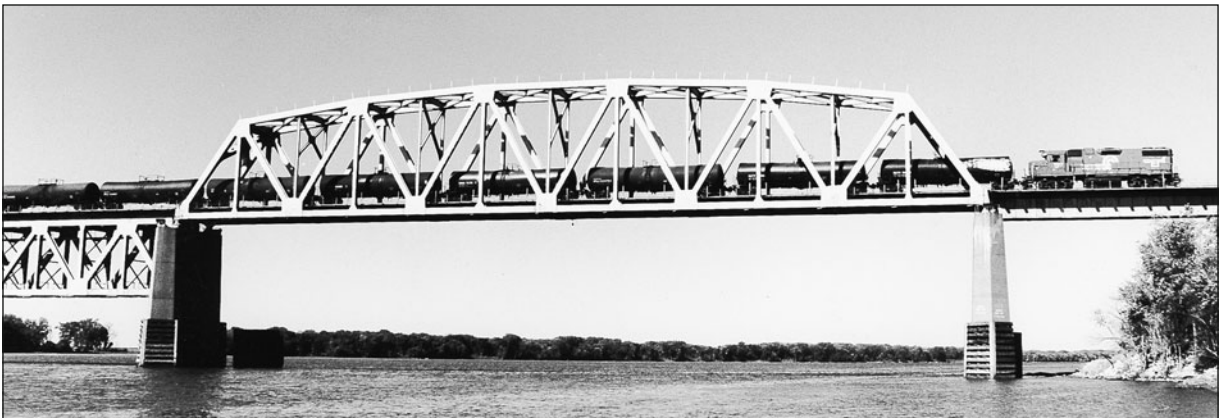
Fig. 5.4. The CB&Q built this high truss bridge across the Mississippi River in 1959–1960 to replace an aged swing bridge. Here, a BN local pulled by a locomotive on loan from Conrail crosses it.
