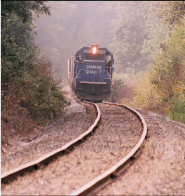
Fig. 1.10. High temperatures, typically 100°F or higher, can produce “sun kinks” in rails, leading to derailments. Here a Conrail train on a branch line in New York state cautiously pulls upgrade on a hot, 99°F, hazy August day with the rails ahead showing many disconcerting oscillations.
