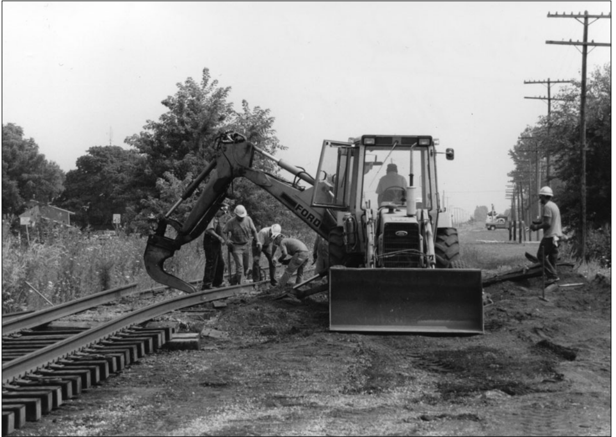
Fig. 5.21. Workers repair a flood-damaged rail line east of New Orleans.
