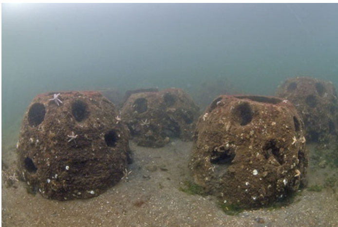
Figure 10.3 Artificial reefs (Reefballs) made with precast concrete near Dreischor in Zeeland (© Reefball International) [18]
