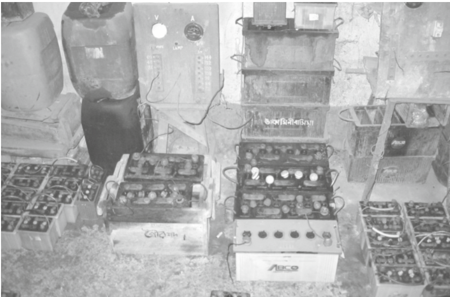
Fig. 1.3 Example of battery types offered in a battery shop
