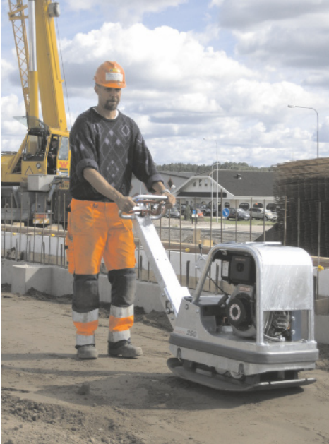
Fig. 3.6 An example of a soil compactor and how it is used (Swepac 2009)
