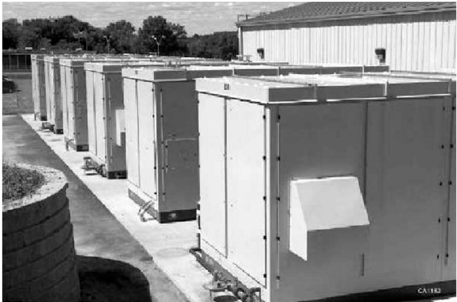
**Figure 1.17(c).** UTC Fuel Cells PC25 6 × 200 kW. (Image courtesy of UTC Power Corporation.)
