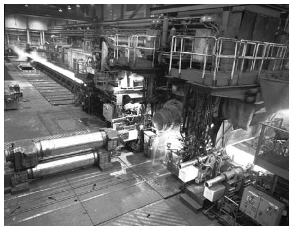
Figure 1: Hot strip mill with replacement roll pair ready.
