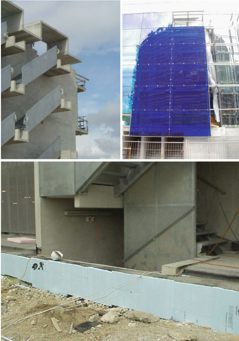
Fig. 10.9 Photographs from the construction site
