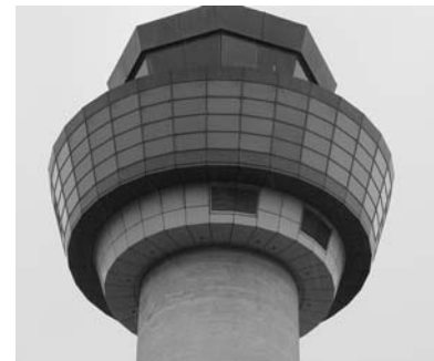
11.2 Air traffic control, part of a complex modern aviation system
