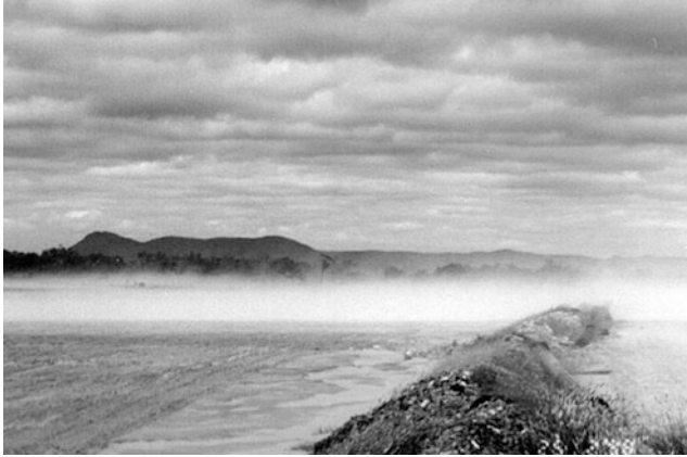
Fig. 8.5. Highly erodable gold mine tailings. A typical windstorm on a new gold mine tailings dam spreading fine particles loaded with heavy metals to the environment.
