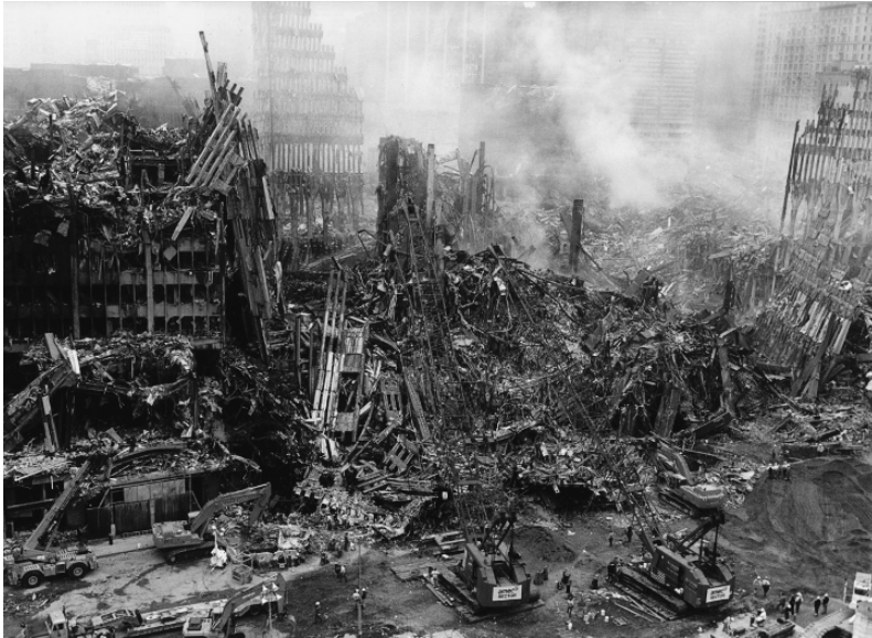
Fig. 7.3 Complicated excavation of Ground Zero showing heavy machinery used (Source: Unknown.)
