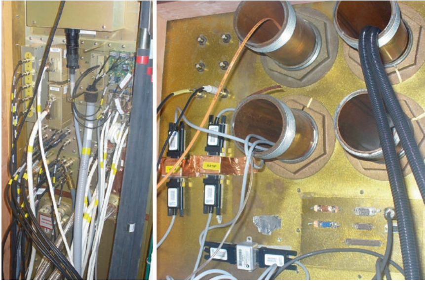
Fig. 5 On the left is the penetration panel that connects the MRI scanner electronics to the magnet hardware. The image on the right is a second penetration panel used for all the additional stimulus/response equipment needed for fMRI
