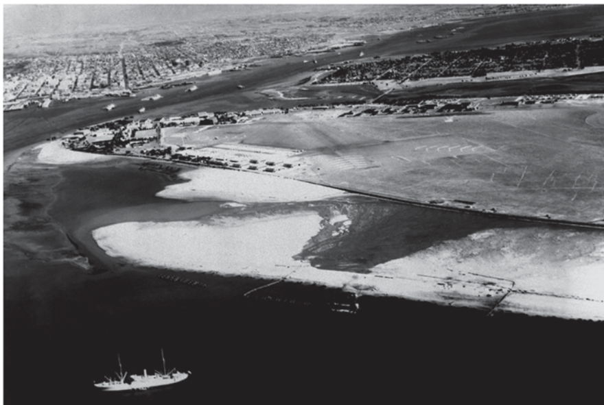
Fig. 5 Filling bay adjacent to NAS North Island in 1936. Viewed east toward downtown San Diego. City of Coronado is to the right, separated from North Island by the Spanish Bight
