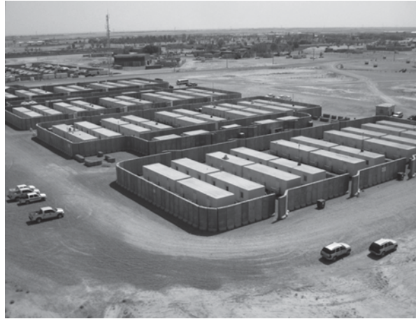
Fig. 2 A living support area (LSA) on COB Speicher comes complete with protective “T-walls,” containerized housing units (CHUs), and community showers and latrines. (Photo courtesy of LTC Joseph P. Henderson, 2010)
