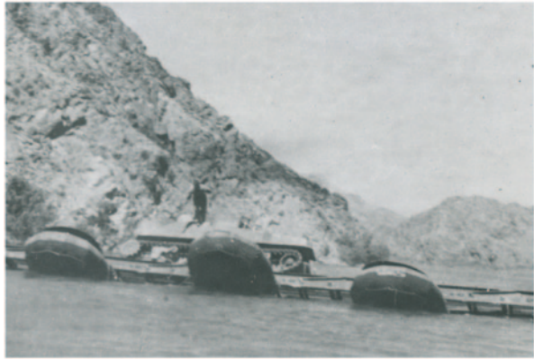
Fig. 4 M-4 Sherman Tank in the midst of an M1 Steel Treadway bridge failure during testing on the Colorado River. (Photo courtesy of the U.S. Army Corps of Engineers)
