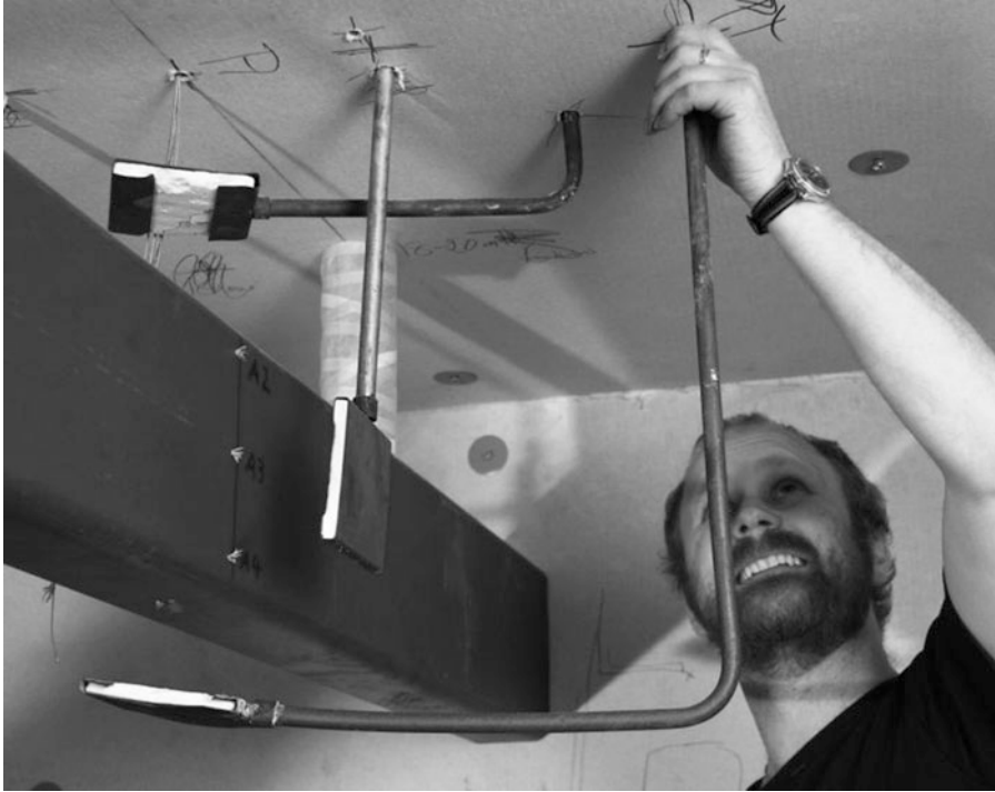
Fig. 34.4 Plate thermometers being mounted around a steel girder for measuring local thermal exposures. Note that the plate thermometers are mounted so that the front
