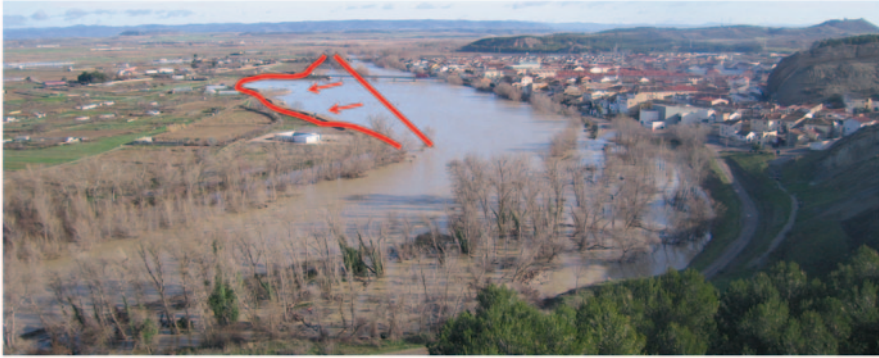
Fig. 9 Aragón River showing the inundation after levee removal from the January 2010 flood near Caparroso
