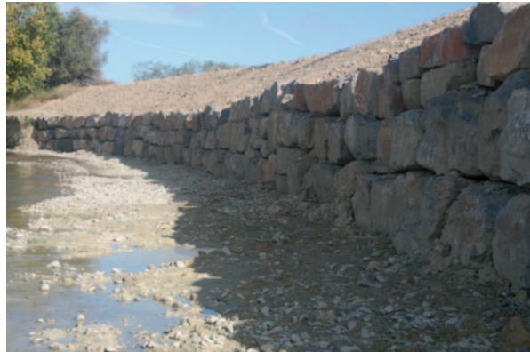
Fig. 4 Embankment built in 2009 (lower Gállego River)
