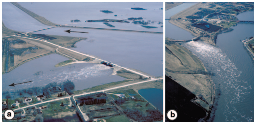
Fig. 8 Photographs during the 1997 Red River flood showing a the split of the flow between the Floodway (flowing toward upper left) and the Red River (flowing towards the lower left), as well as the Floodway Inlet Control Structure (centre right) and the flood zone (top, beyond dyke), and b the Floodway Outlet Structure and confluence of the Floodway (entering from left) and Red River (see Fig. 2 for locations). Note, in b the entire flow of the river is confined within the river channel in contrast to the situation upstream of the Floodway inlet. Photographs taken 9 May 1997
