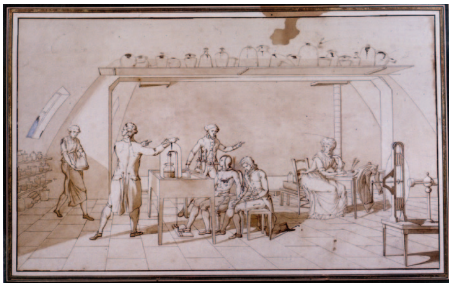
Fig. 12.5 Drawing by Marie-Anne Lavoisier of an experiment on oxygen consumption in a subject while exercising. The expired gas is apparently being collected by mercury displacement. The subject's right foot is on a pedal that allows him to do mechanical work. Anne-Marie Lavoisier is on the extreme right . See text for details. From [6]
