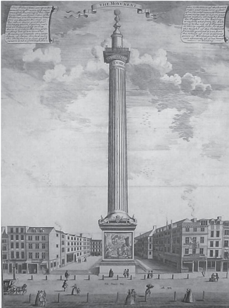
Fig. 6.5 Monument to the Great Fire of London of 1666 which still stands. It was designed by Hooke and Christopher Wren and also served as a zenith telescope. By permission of the London Metropolitan Archives, City of London
