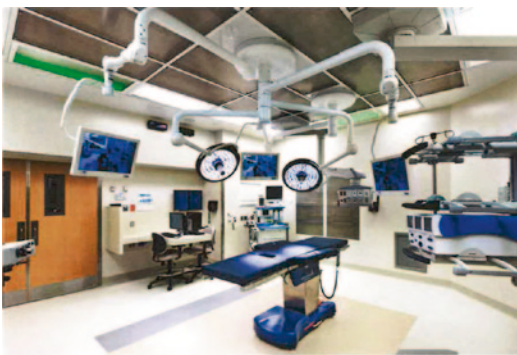
Fig. 1.4 MIS general OR. ORs at specific hospitals are designed to a common standard. Equipment is always integrated within the standard work environments, and interfaces remain consistent throughout the ORs. This photograph illustrates lighting requirements, including ceiling lights, spot LED lights, and green light for dimmed environments. Diffusers in the center of the room for laminar airflow are also seen
