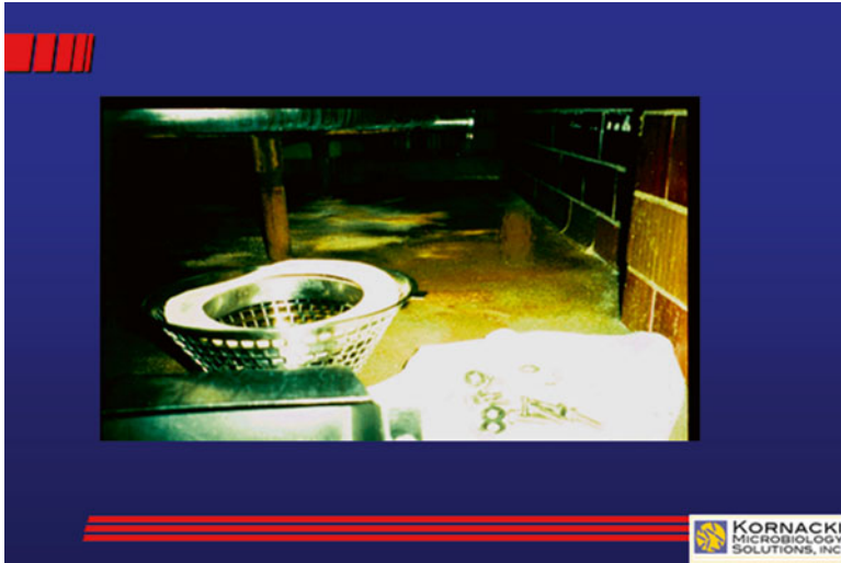
Fig. 6 Hammer mill placed in unclean area after wet cleaning
