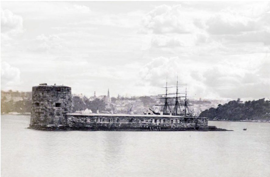
Fig. 5.3 Pinchgut [i.e. Fort Denison], Sydney undated [pre-1885], Sydney Harbour, NSW. Photographer unknown/Source: National Archives of Australia
