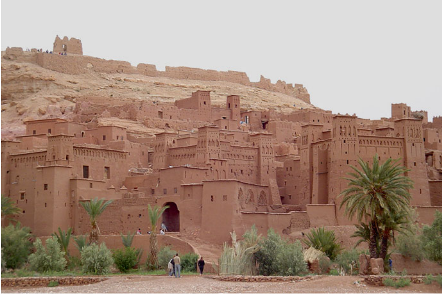
Fig. 5.4 The fragile and vulnerable earthen World Heritage Site of Ksar Ait ben Haddou, Maroc. Photograph J. Hurd
