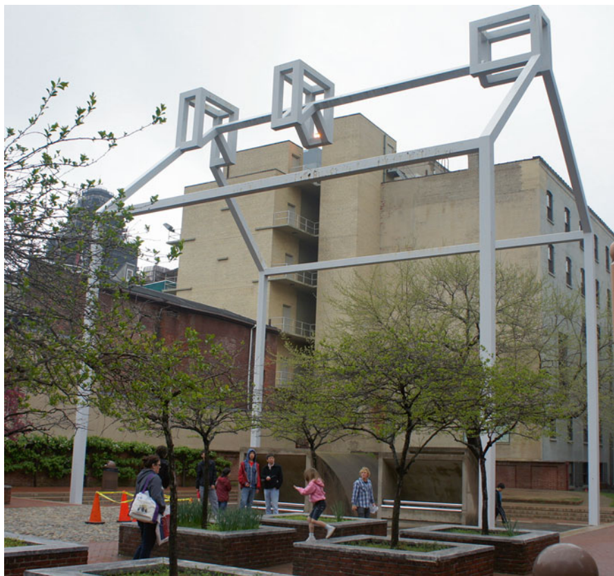
Fig. 7.8 The Venturi and Rausch designed ‘ghost house’ (1976) Franklin Court, above the archaeological remains of Benjamin Franklin’s demolished residence, Philadelphia, USA. Photograph by the author 2011
