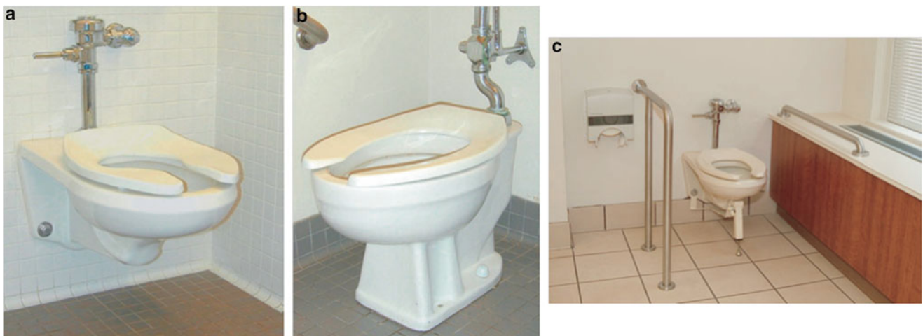
FIG. 8. (a) Wall-mounted commode. (b) Pedestal commode. (c) Handrails and adequate space around the commode (Courtesy of Bariatric and Metabolic Institute, Cleveland Clinic, Cleveland, OH)
