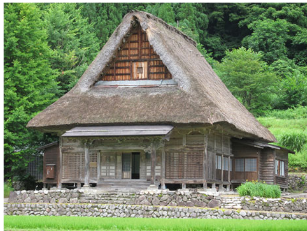
Fig. 3.2 A traditional style of Japanese architecture with a thatched roof
