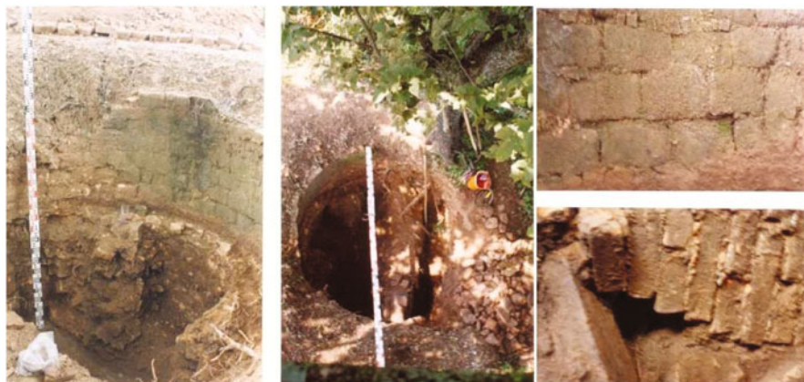
Fig. 3.3 Brickworks in the Hacienda Tune. (Photography by Angélica Suaza; taken by Suaza 2007, p. 138)
