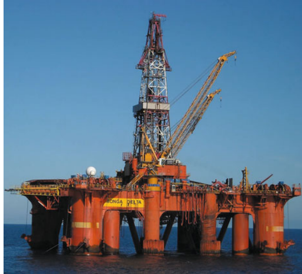
Fig. 13.1 The semi-submersible rig Songa Delta operating in the North Sea
