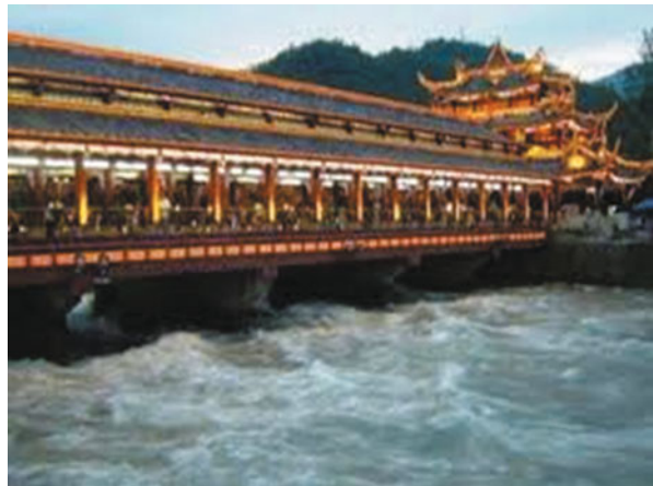
Fig. 7.3 Dujiangyan dam in China. For details see the source “Images for Dujiangyan Dam” at https://www.google.co.in/search?q=Dujangyan+Dam+pictures
