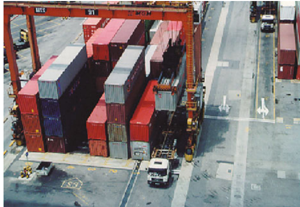
Fig. 1.5 Six rows of stored containers and seventh (rightmost) row used as a lane for truck passage in a storage block. You can see the yard crane (YC) lowering a container retrieved from storage onto an internal truck (IT)
