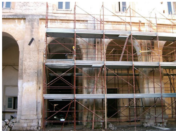
Fig. 5.2 Series of star vaults in a building in Lecce (Southern Italy)
