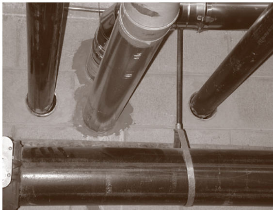
Fig. 11.63 Examples of sealed pipe and duct penetrations
