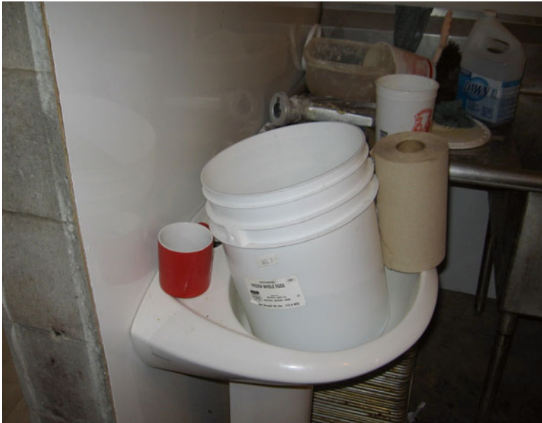
Fig. 12.9 Employee handwashing station
