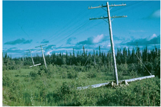
Fig. 5.9 Tilting of a line of poles in a bog is also caused by freezing and thawing, Yukon region, Alaska. The cross-poles at the base are to minimize the effect. Photograph by T.L. Pewe, U.S. Geological Survey
