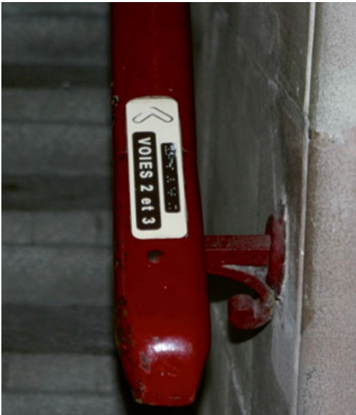
Fig. 23.4 Perceptible information. Perceptible information can be achieved by the use of high-contrast, directional, and tactile information
