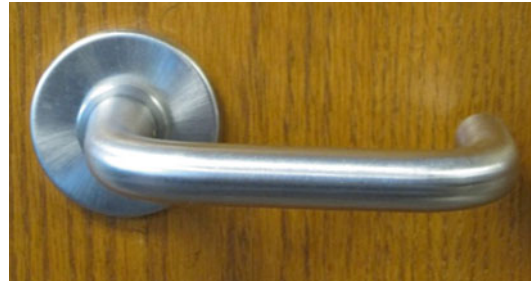
Fig. 23.2 Flexibility. Flexibility in use permits alternative methods of use including open hand, closed fist, or elbow
