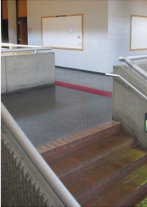
Fig. 23.5 Tolerance for error. Tolerance for error can take on many forms such as the use of tactile and visually contrasting floor materials to indicate the location of intersections and stairways
