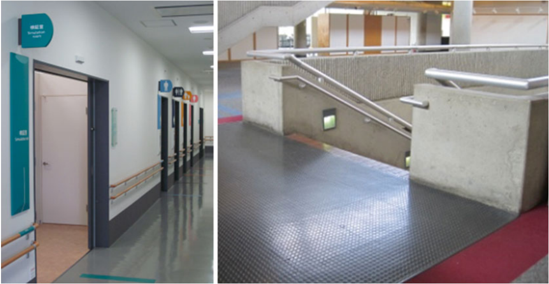
Fig. 23.9 Corridor. Redundant and multisensory way-finding systems including color changes in signs and floors at different rooms as well as tactile information on walls, floors, and handrails facilitate moving around the work environment
