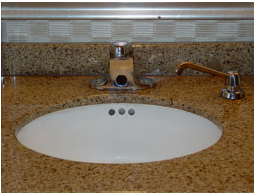
Fig. 23.6 Low physical effort. Low physical effort is afforded by an electronic faucet that requires no physical force to operate
