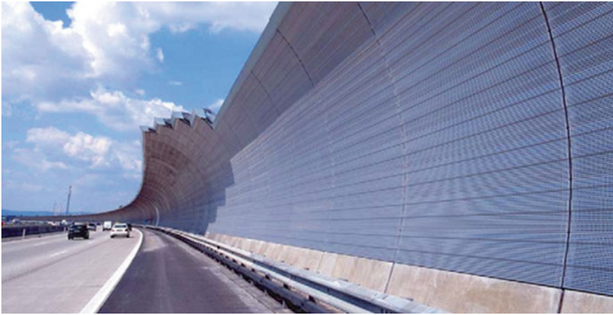
[67] Vienna, Austria Steel highway noise barrier
