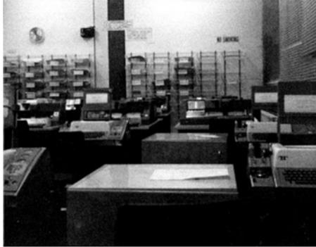
The machines in the foreground are teletypes. They printed onto paper (in capital letters only) at 110 baud. I can type faster than a teletype can show what I'm typing.
