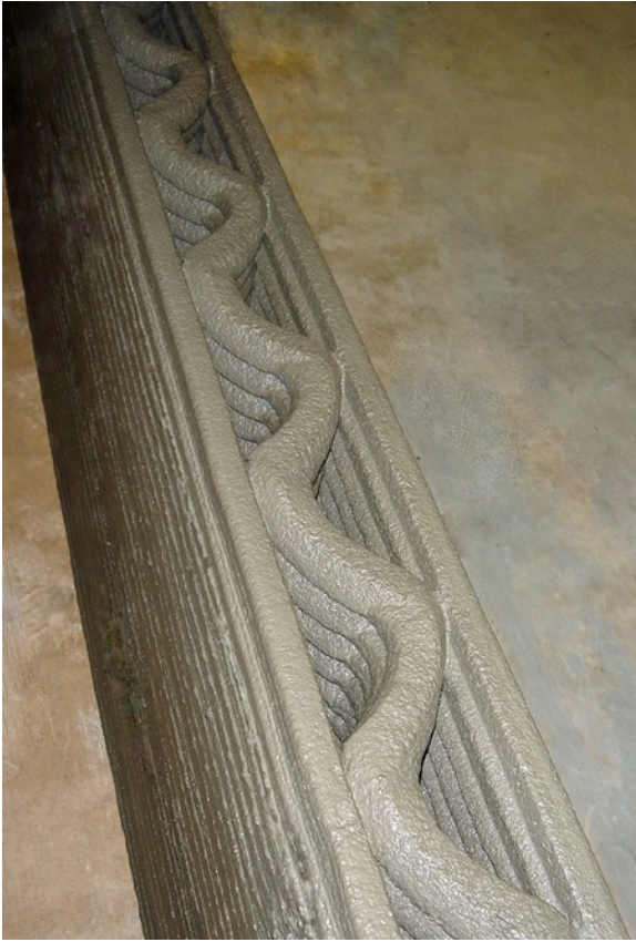
Figure 14-1. A section of 3D printed concrete wall. Courtesy of Contour Crafting
