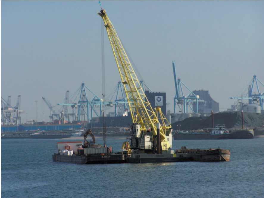
Fig. 9.2 Excavations in the Yangtze harbour basin, Rotterdam. A Mesolithic occupation layer at 20 m below the water surface is being sampled by means of a special crane. Samples are packed in large white bags, before being wet-sieved. For the first time, Mesolithic occupation remains were uncovered from a submerged landscape under relatively controlled conditions. (Photo by B. Smit, Rijksdienst voor het Cultureel Erfgoed, courtesy of the Port of Rotterdam)
