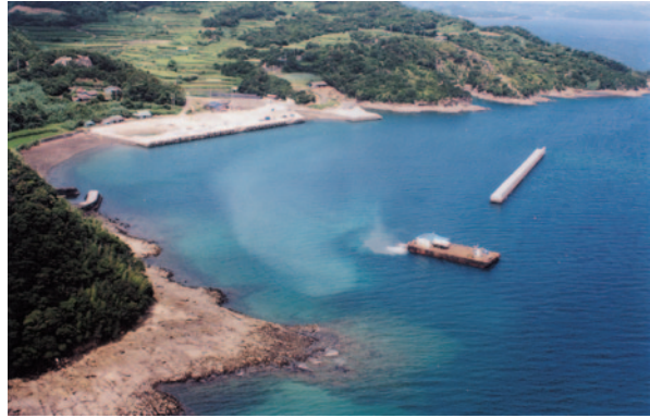
Fig. 15.3 A photograph showing Tokonami harbor excavation. (Photo courtesy of Asahi Shinbun)
