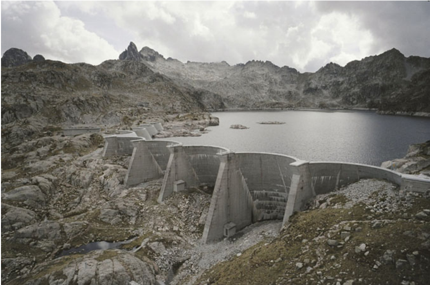
Fig. 1 Aerial view of Migouélou dam and lake, © EDF, Gilles De Fayet
