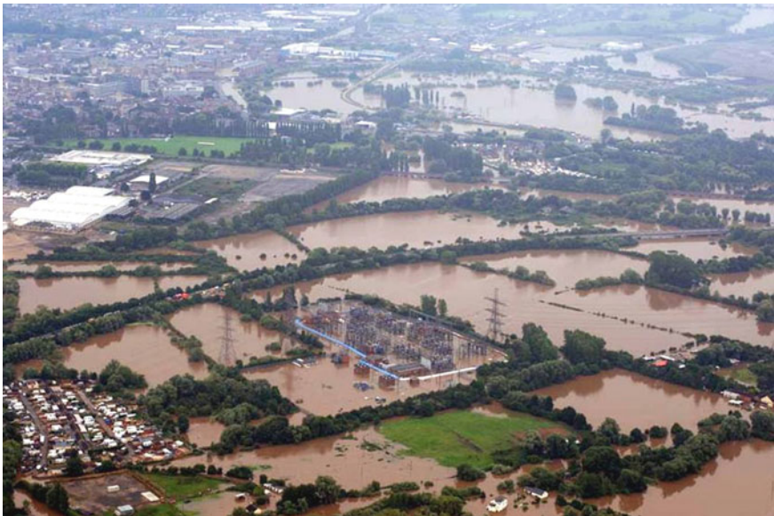
Fig. 8 Example of flooding in Gloucestershire, UK 400 kV substation
