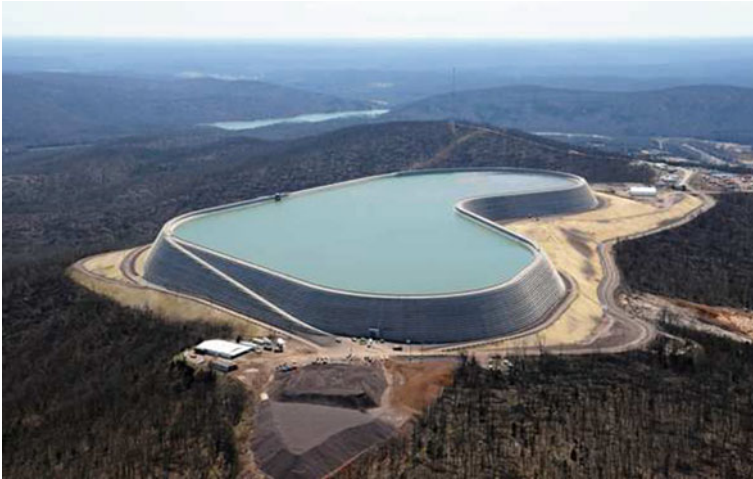
Fig. 7 Taum Sauk 450 MW custom pumped hydro storage system in Missouri
