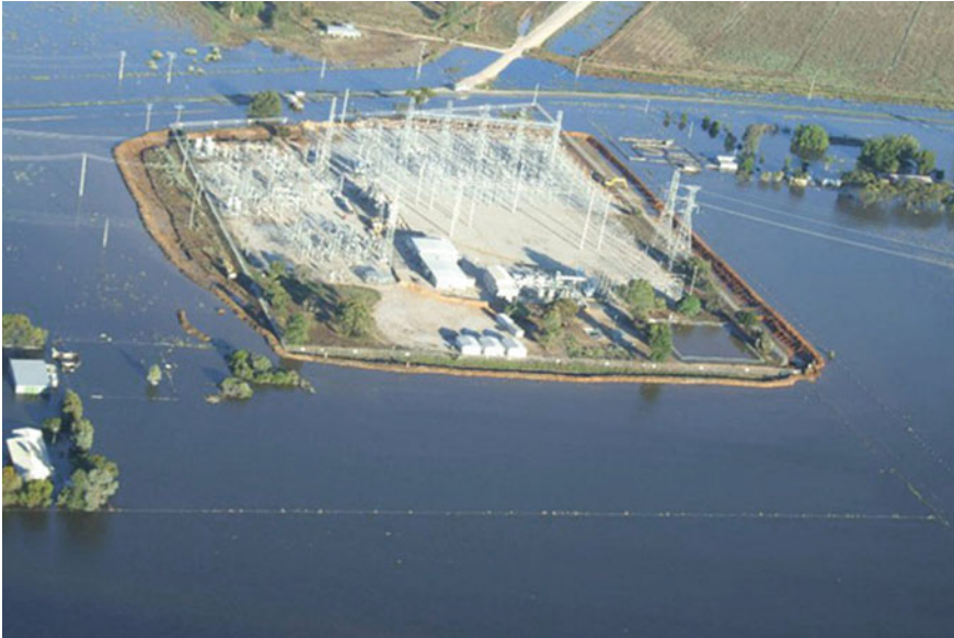
Fig. 9 Aerial photo of Kerang Substation in Victoria in January 2011
