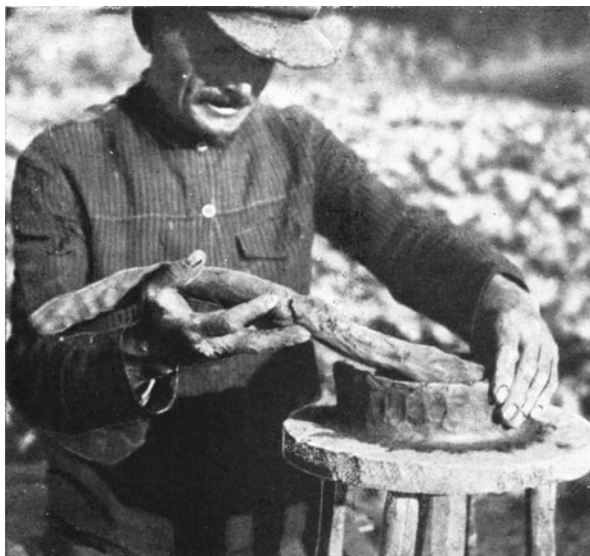
Fig. 5.6 Village of Zamosze, commune of Wołkołata (now Zamošša, Belarus). The potter attaches a second coil of ceramic paste. Photo: Włodzimierz Hołubowicz 1937–1939. After Hołubowicz (1950): photo 30
