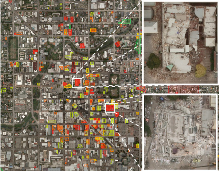
Fig. 8 Results of the crowd-contributed damage outlines and highlights of two destroyed buildings. Red = completely destroyed, orange = heavy damage, yellow = light damage
