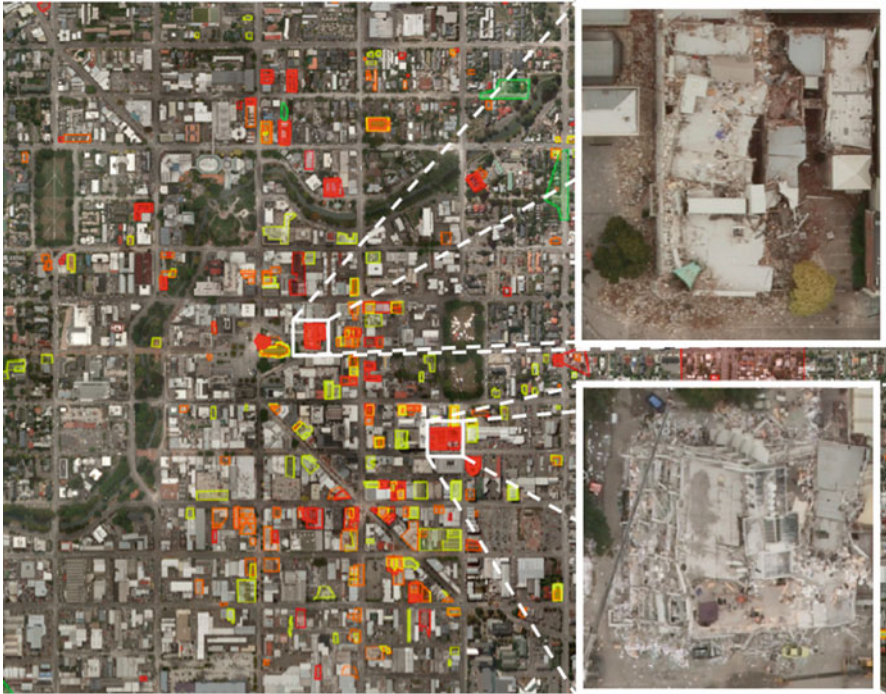
Fig. 8 Results of the crowd-contributed damage outlines and highlights of two destroyed buildings. Red = completely destroyed, orange = heavy damage, yellow = light damage
