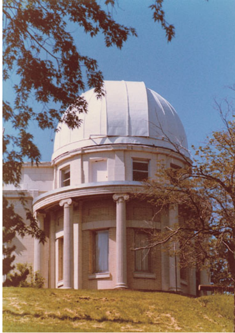
Fig. 10.4 A charming example of the classical domed observatory. The most aesthetic-looking of the various types of telescope shelters, it offers the greatest protection from wind and stray light. However, it also has the most limited view of the sky (due to its narrow slit) and is the most costly of all the types of housings. Photo by Sharon Mullaney
