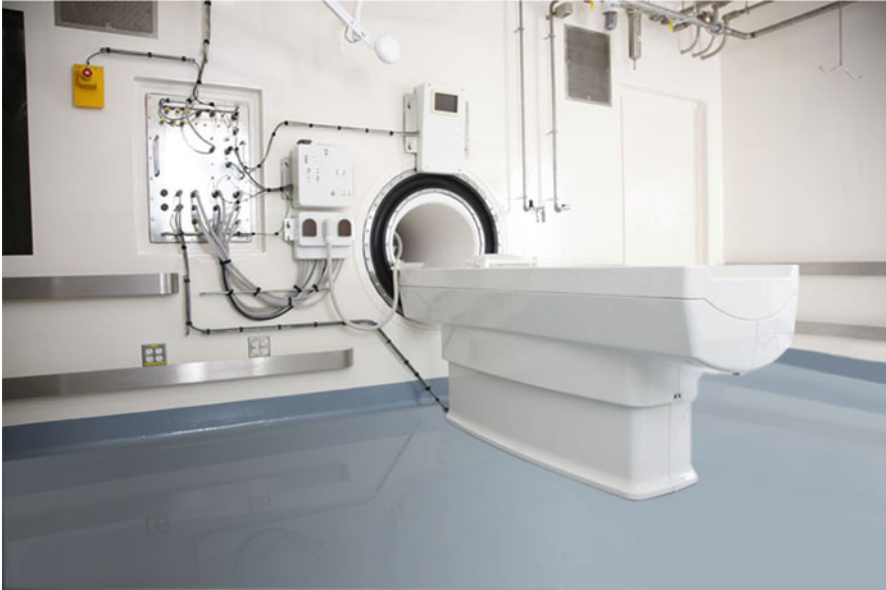
Fig. 10.7 High-containment side of the magnetic resonance imaging room at the National Institute of Allergy and Infectious Diseases Integrated Research Facility at Fort Detrick, MD. The black ring around the bore entrance is a gasket that seals the connection between the containment tube and the barrier wall
