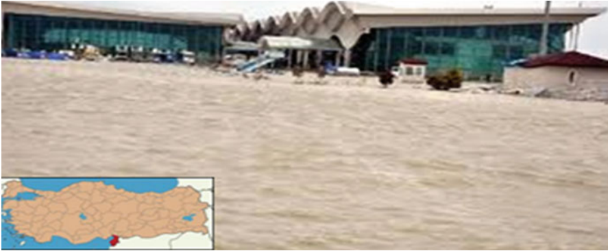
Fig. 22.5 Flood in Hatay airport ( bottom left : place in Turkey) [4]
