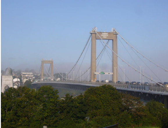
Fig. 1 The Tamar suspension bridge
