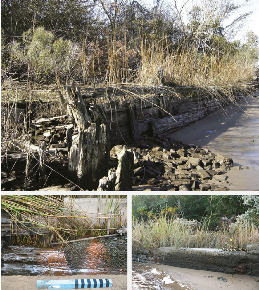
Fig. 12.3 Evidence of reuse can be seen among the abandoned remains. Top The bow of Bulkhead Tug in the foreground, which is filled with brick and rock debris, abuts the Bulkhead Barge, creating a bulkhead for the railway to the north. A concrete wall connects two barges, creating a bulkhead. The concrete wall built into the structure and fabric of the Bulkhead Barge ( bottom left ) and the concrete wall extending north out of the Bulkhead Barge toward Barge 3 ( bottom right ). (Images by Sami K. Seeb)
