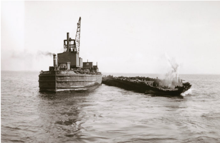
Fig. 4.4 The crew of Cobourg (left) sets off a dynamite charge in the stern of Stormount at the Nine Mile Point Ship Graveyard, September 30, 1937. The thin wooden cross amidst the spray suspends the detonator wire. (LAC, Department of Transport fonds, file no. 8308-128, e010963487)
