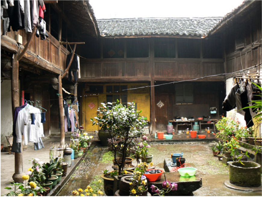
Fig. 5.4 The courtyard of a large hotel, Hotel Chengchengchang. (Photo by author)
