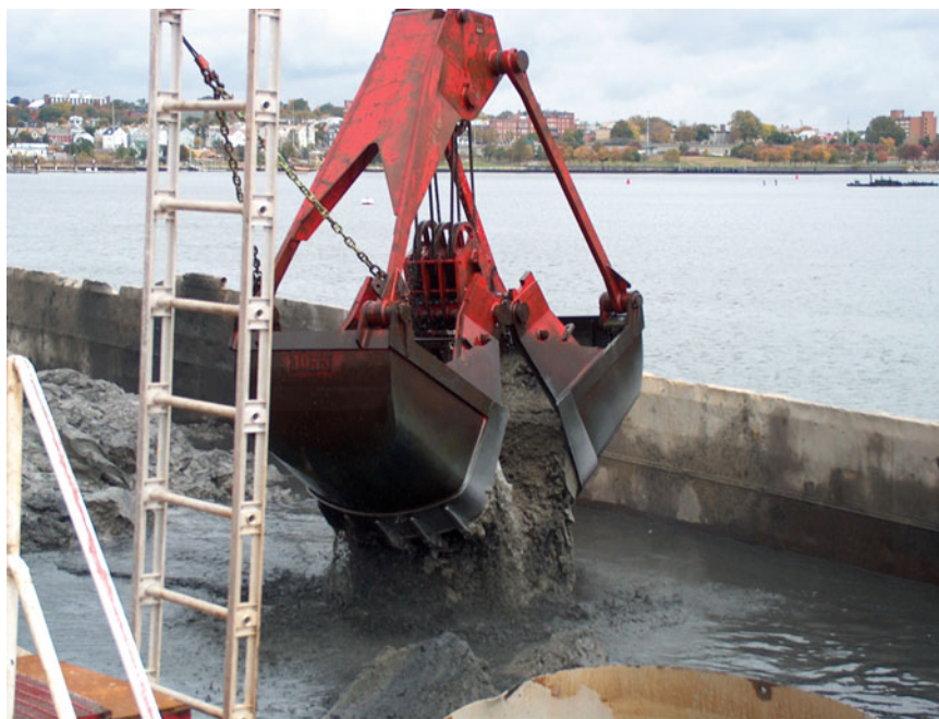
Figure 6.1. Navigation channel dredging using a clamshell (or bucket) mechanical dredge.
