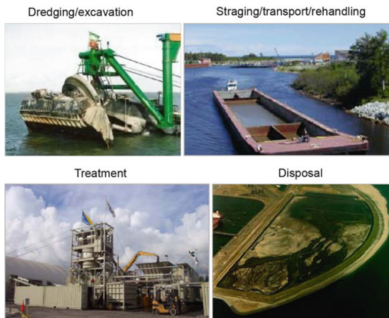
Figure 13.1. Components of a sediment removal remedy.
